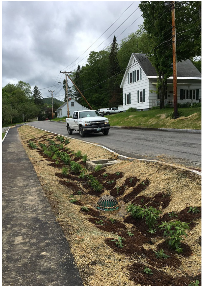
Above: A recently installed rain garden on Saranac Street as part of the River District redevelopment efforts. Rain gardens absorb stormwater runoff, filter pollutants, and encourage infiltration, protecting the water quality of the River while also providing beauty and pollinator habitat.
